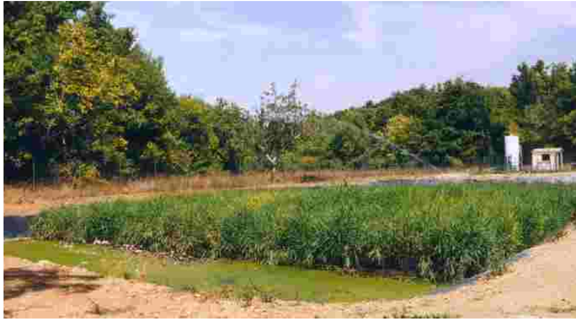
Horizontal subsurface flow system (used as a tertiary treatment)
