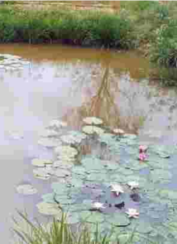
Detail of a Surface Freeflow System for a wine-producing firm (Siena, Italy)
