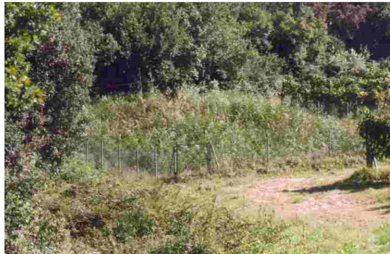
Horizontal subsurface flow system (Siena, Italy)
