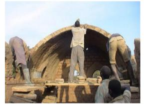
straw, with optimal dimensions to stick to the fresh mortar near the top of the vault; the use of oil drums as temporary supports for forming window and door arches; the use of plastic sheeting over the roof, covered by a final waterproof rendering to protect it from solar degradation, and to reduce the annual maintenance load for the roof
