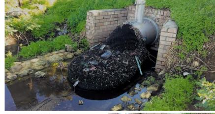
The nets have been placed on the outlet of two drainage pipes, which are located between residential areas and natural areas. This allows the nets to capture the gross pollutants carried by storm water runoff of the local road network before those pollutants are discharged and contaminate the natural environment at the downstream end of the outlet area. This ensures that the habitat of the local wildlife is protected and minimizes the risk of wildlife being caught in the nets.
