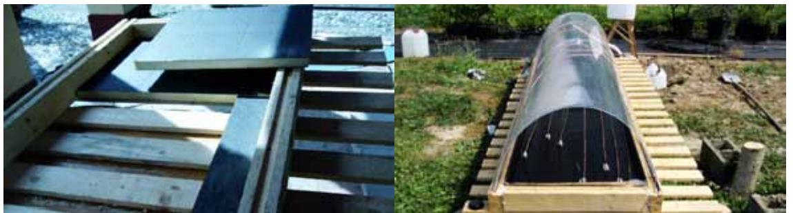
Figure 2. Building steps of the solar still, employing economic and easily available materials
