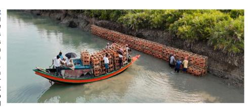
WWF-India, through the Sundarbans Delta Program, World Wide Fund for Nature has placed thousands of terracotta rings in human-inhabited as well as forested areas of the Sundarban to secure the shoreline. When the high tide comes in, bearing silt, the rings trap the silt, preventing erosion and stabilising elevation.
