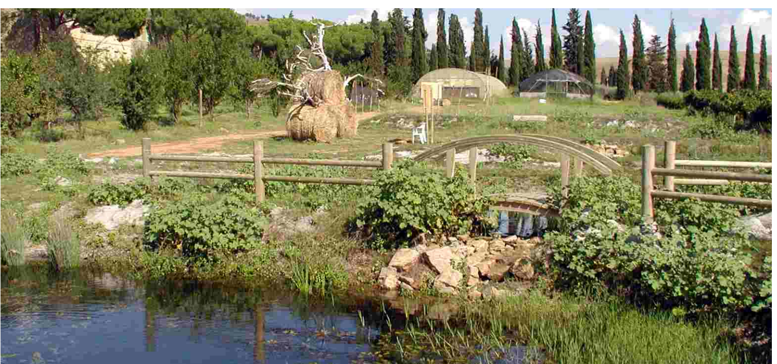
Surface free flow system (FWS) for the treatment and collection of rainwater to be re-used (Grosseto, Italy)
