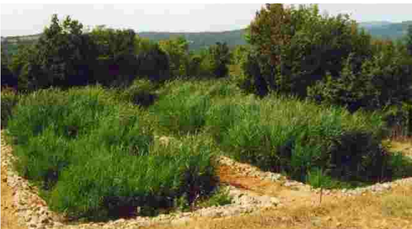
Horizontal subsurface flow system (Siena, Italy)
