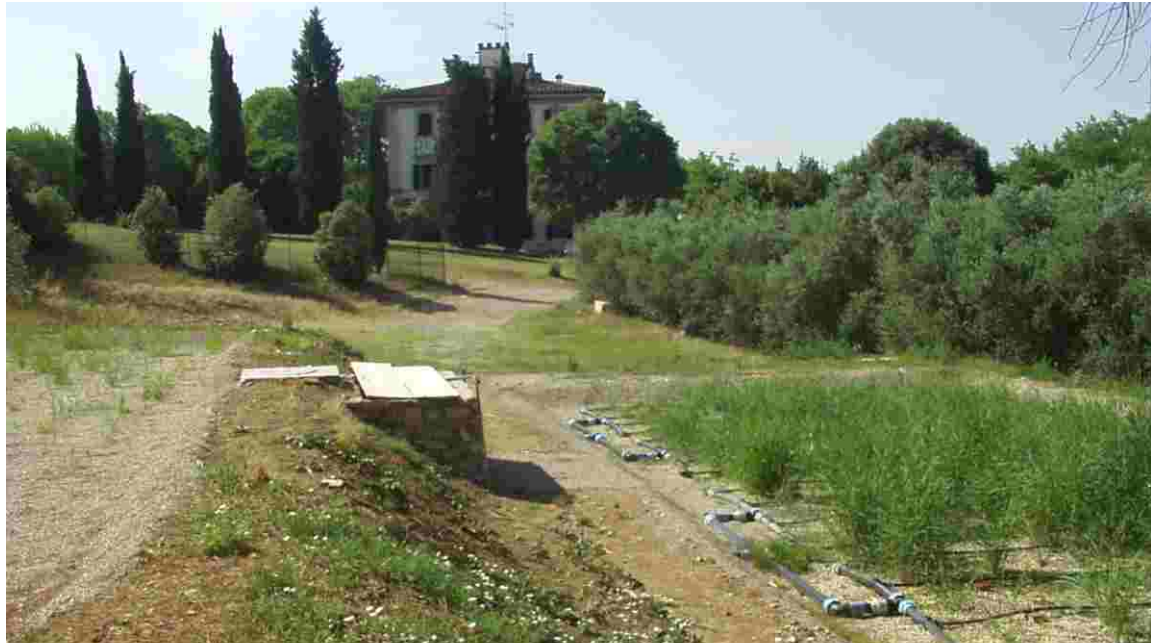
Detail of a multi-stage system consisting of a horizontal subsurface flow system (right) and a vertical one (left) at the service of a tourist structure - 140 equivalent inhabitants (Florence, Italy)
