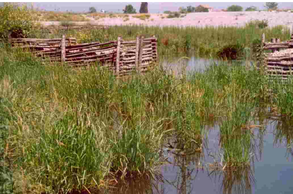
Free water system (used as a tertiary treatment)
