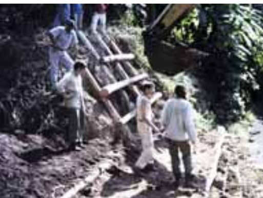
Construction site in León, Nicaragua 2004
