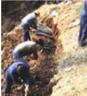
A typical example of stabilization – “brushlayer” (Tuscany region, 2000-2001)
