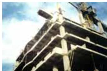
**Cantilever floor slabs**, which replace edge beams in architectural solutions where balconies, loggias or other housing space out of column span are required and which are connected only to two columns (as a cantilever) and their height and length correspond to floor slabs near which they are erected, while their maximal width is limited on 1/3 of the longitudinal span. They are waffled and can be with or without concrete ceiling.
