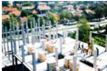
**Floor slabs** cover space between columns and can be manufactured with or without concrete ceiling, as one-piece (spans until 3.6 x 4.8 m) or multi-pieces aiming to adapt dimension for transportation and erection (ceilings made for the span 9.0 x 9.0 m are constructed from nine standard elements); the marginal girder and waffle web height is 20-40 cm (depending on column span between which space is covered), floor slab depth between coffer webs is 4-6 cm, and the ceiling one is 3cm.
